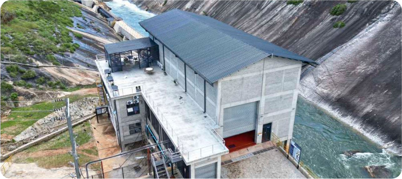
Great Zimbabwe Hydro, completed in 2025, currently generating 5.4MW.
