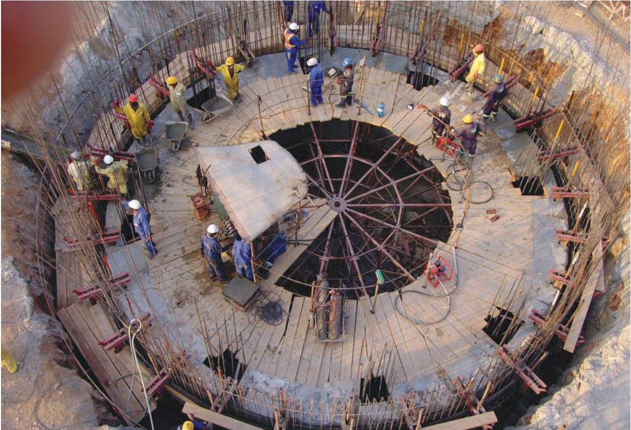
Construction work in progress
