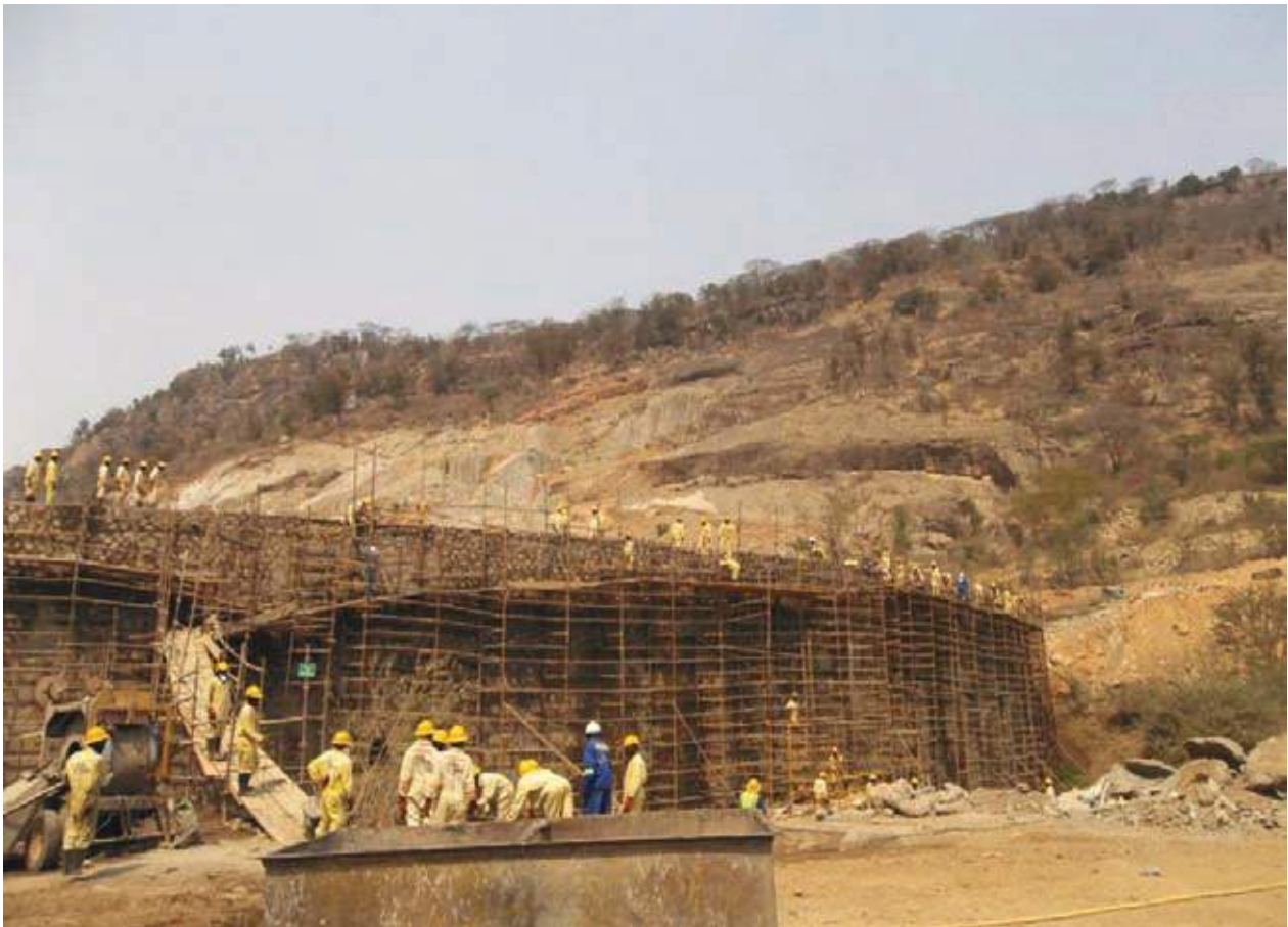
Tokwe-Mukorsi Dam under construction
