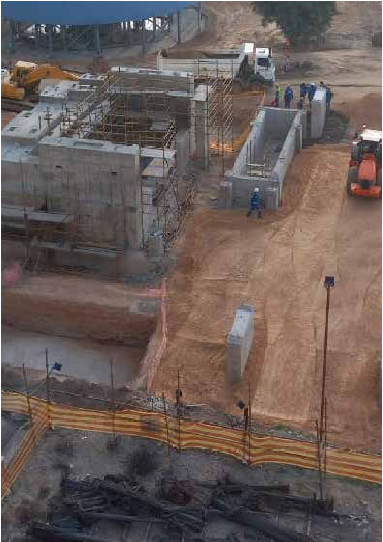
Secondary Millings Earthworks and Civils
