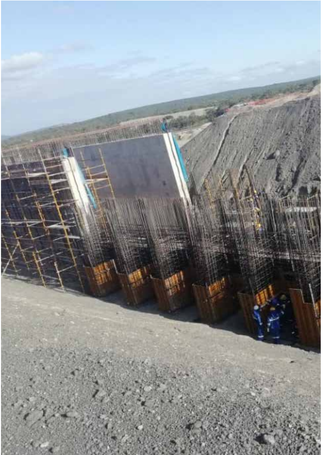
Dome Tunnel Civils
