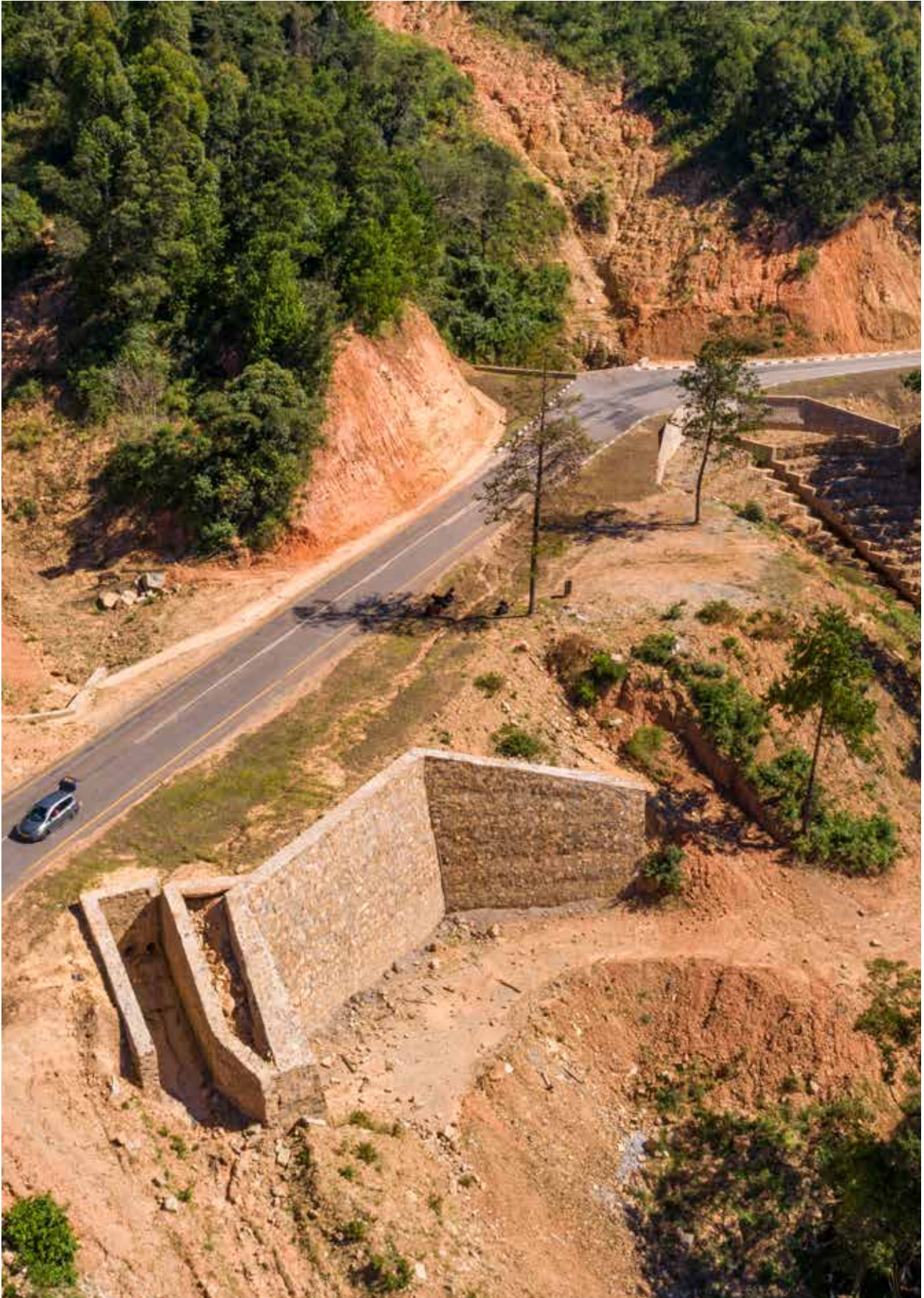
Skyline Chimanimani Road Works
